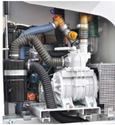
Vacuum pump configuration
